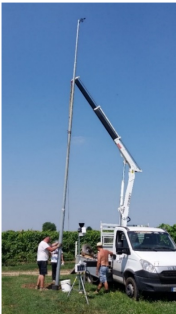
Fig. 10a Installation of the anemometer pole.
