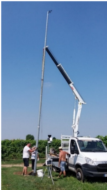
Fig. 10a Installation of the anemometer pole.
