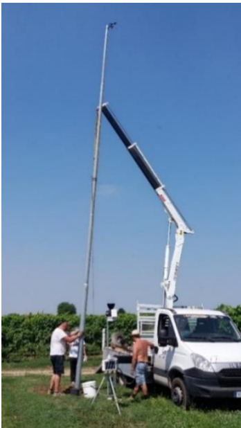
Fig. 10a Installation of the anemometer pole.
